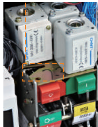
Figure 82.NA1 instal the locking system
