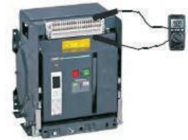
Figure 56. Inspection of secondary circuit
