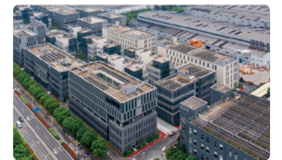
Power T&D Shanghai Factory China Main Products: Power Transformer, GIS, MV and LV Switchgear, HGIS, HV Circuit Breaker, Disconnecter
