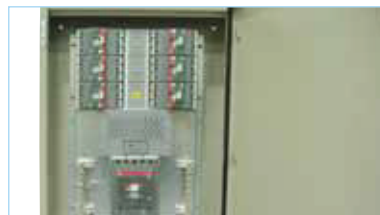
MCCB Pan Assembly Panel Board
