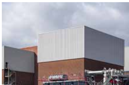
Waste Management Facility @ Tuas
